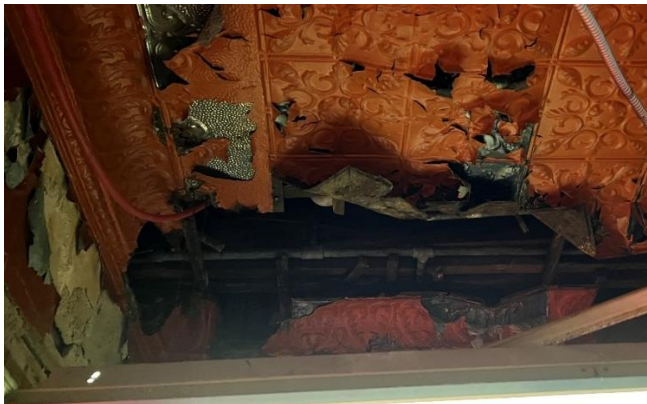
Typical ceiling condition
