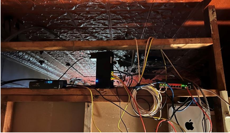
Wall above dropped ceiling at closet.
