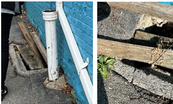
Front lightwell condition
